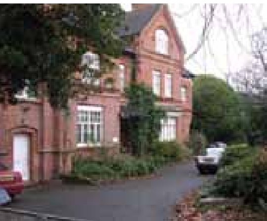
Opportunity to improve the appearance of the driveway
