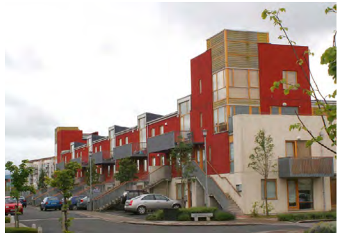
BH5 includes houses above houses – such as these visited by the Neighbourhood Team at Cherry Orchard in Dublin
