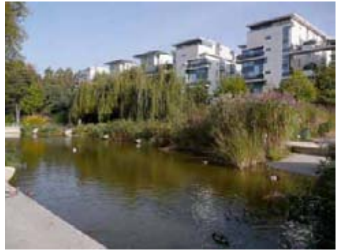
Development adjacent to Parc Bercy shows a strong building frontage, whilst allowing for views of the park
