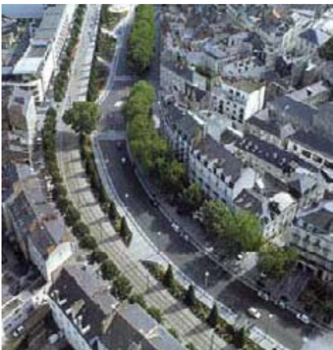
Thurlow Street will include space for all modes of movement, including public transport
