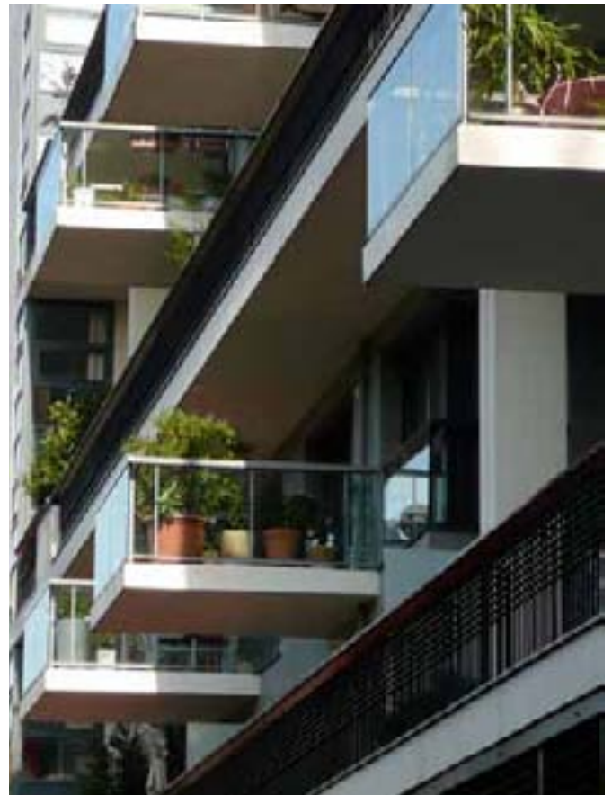
Balconies should be of a good useable size
