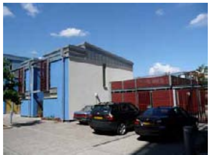
Refuse storage should be convenient, easy to access and unobtrusive
