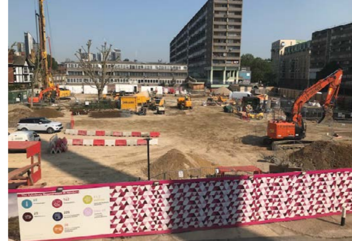
Plot 18 progress on site
