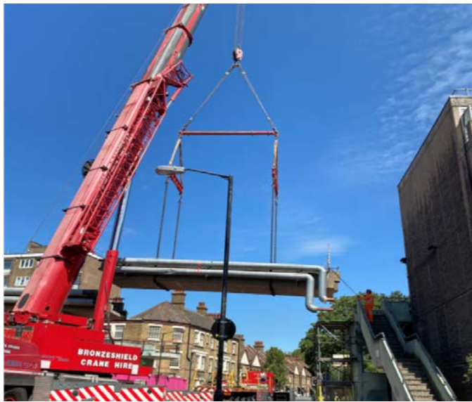
Portland Street bridge removal
