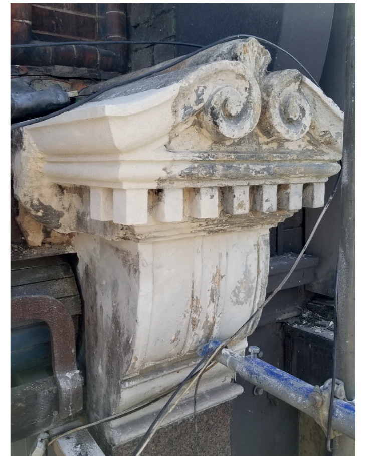
restoration works to the Portland stone capitals
