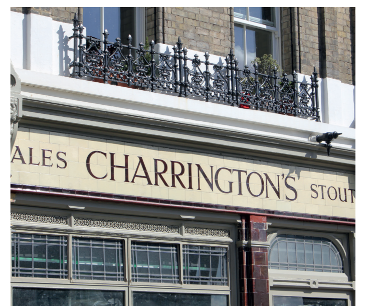
replicating the fascia tiles and decoration works to the lead windows
