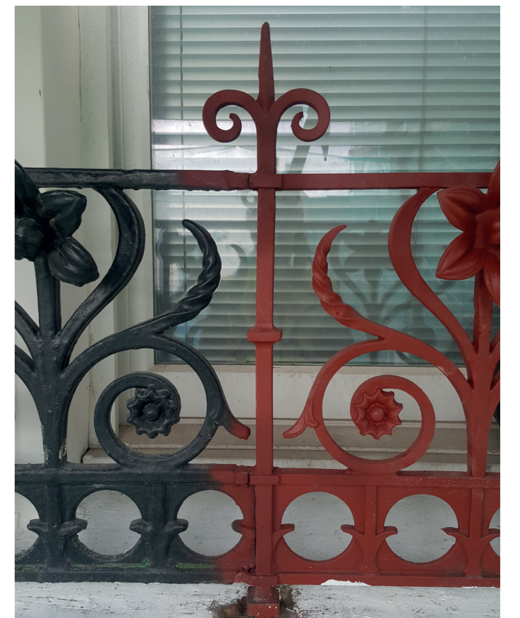
restoration works to the missing decorative cast ironwork
