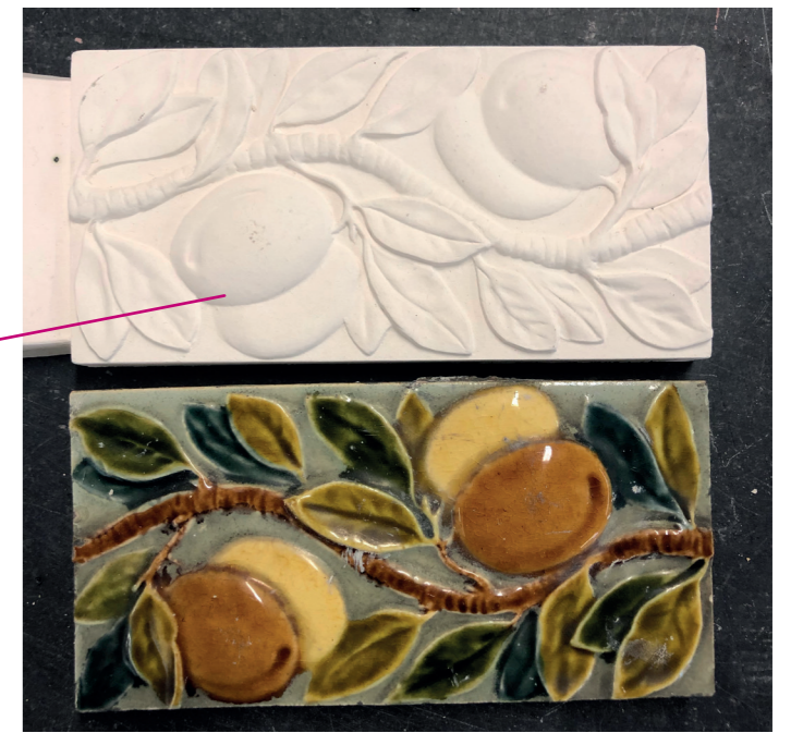
replicating the frieze tiles and decoration works to the fascia
