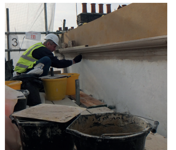
restoration works to the upper cornice
