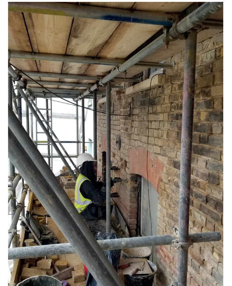
restoration works to the brickwork
