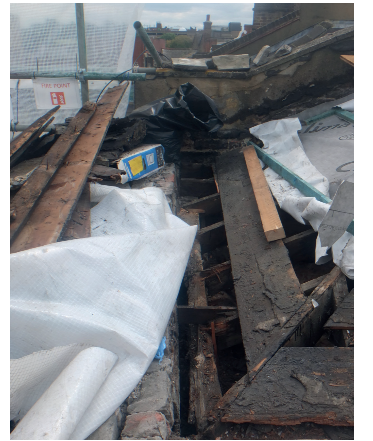
exposing the roof condition behind the parapet
