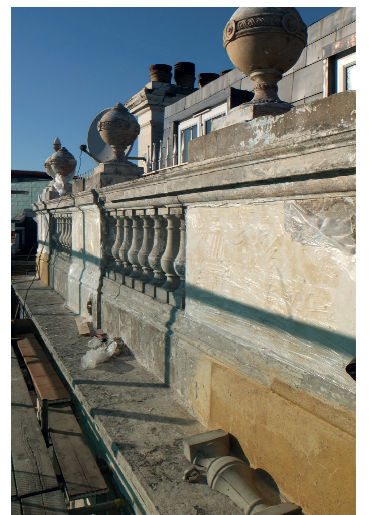
restoration and redecoration works to the parapet balustrade finials
