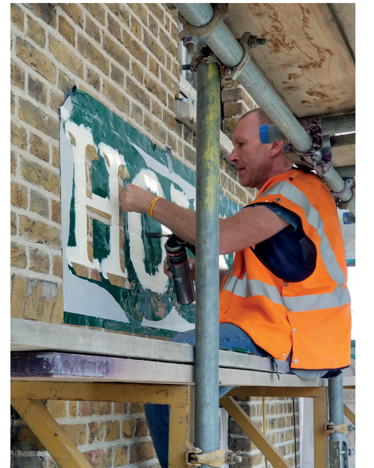
new signage using handpainted stencil graphics directly onto the brickwork
