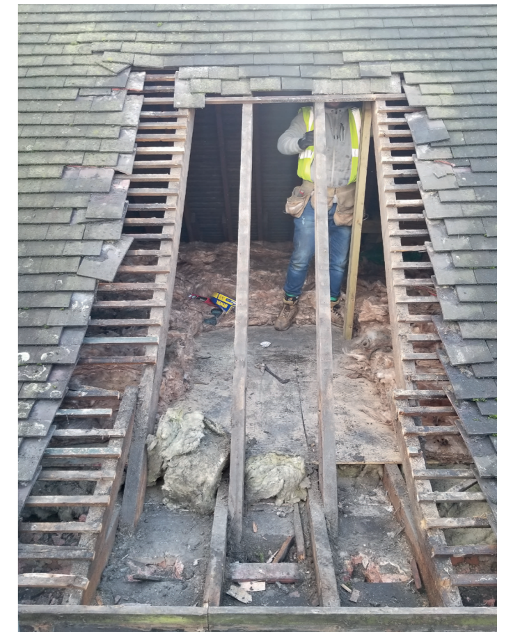
restoration works to the pitch roof dormer
