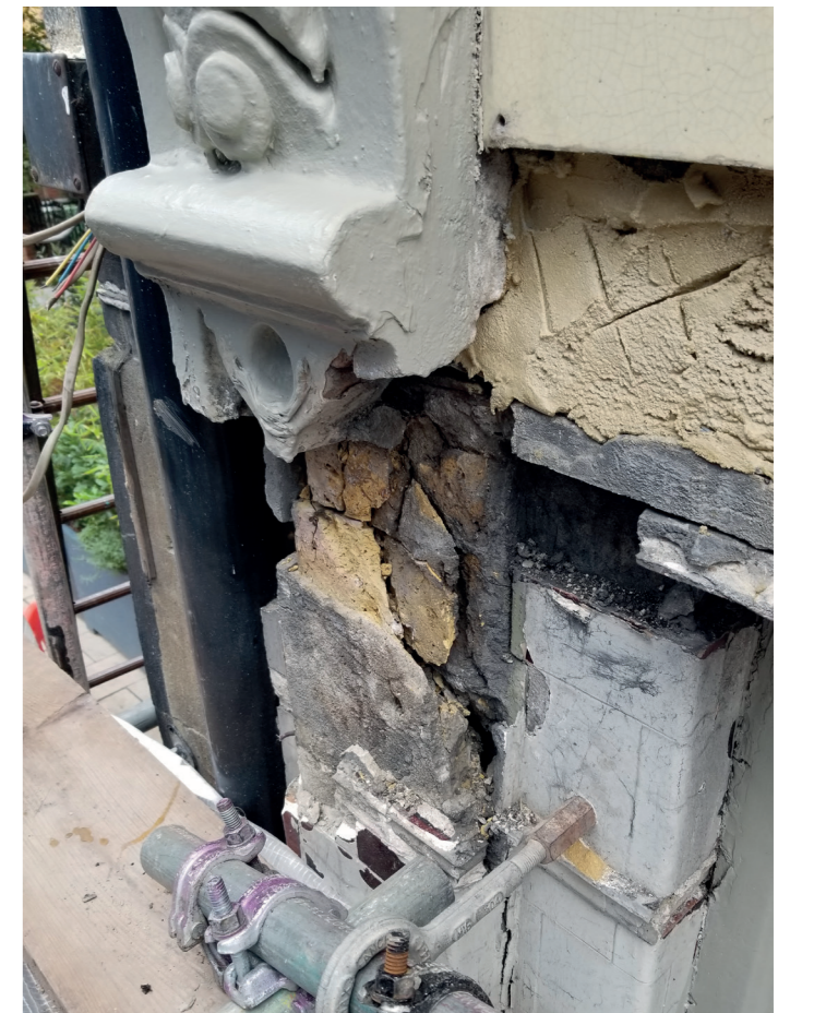
investigation works to a missing pilaster head
