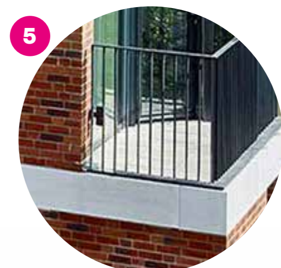
5 White Concrete Lintels & Balcony Fascia Panels
