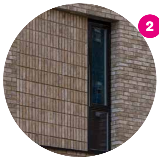
2 Triple stacked vertical brick banding.
