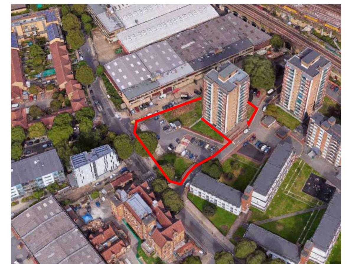
4. Aerial view to the site
