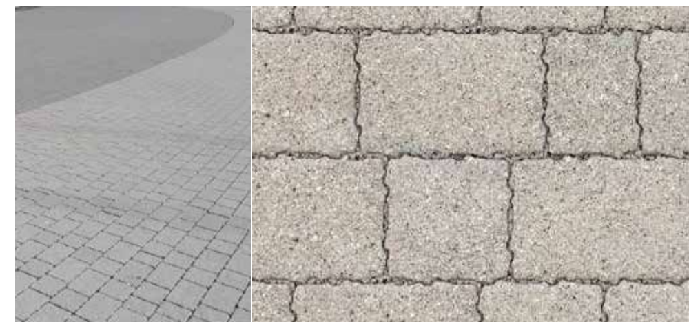
Porous block paving to the pedestrian entrance area from Galleywall Road, and to the disabled parking bays
