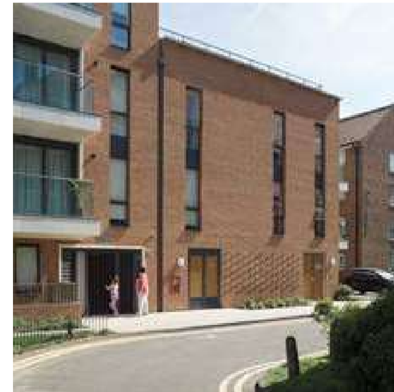
Masterman House garages / Lomond Grove SE5
