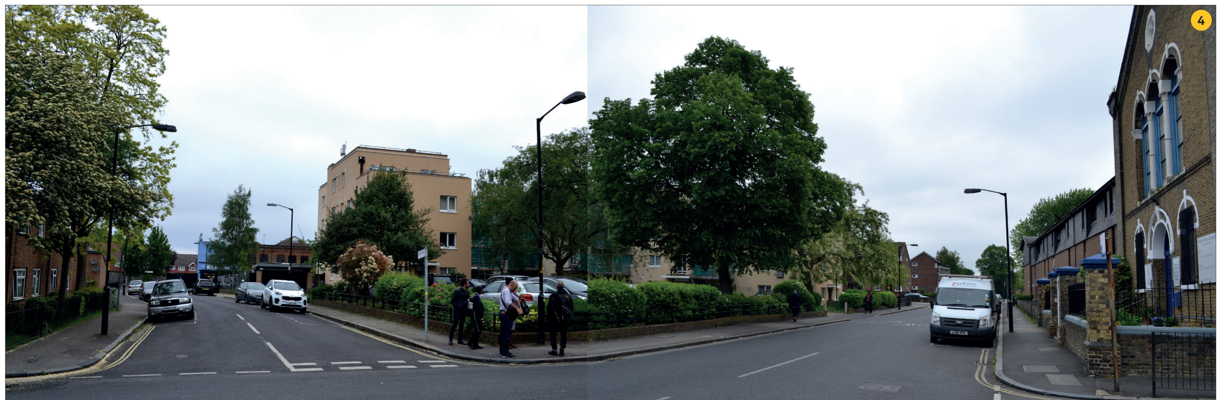
▲ View of site looking north from Heaton Road
