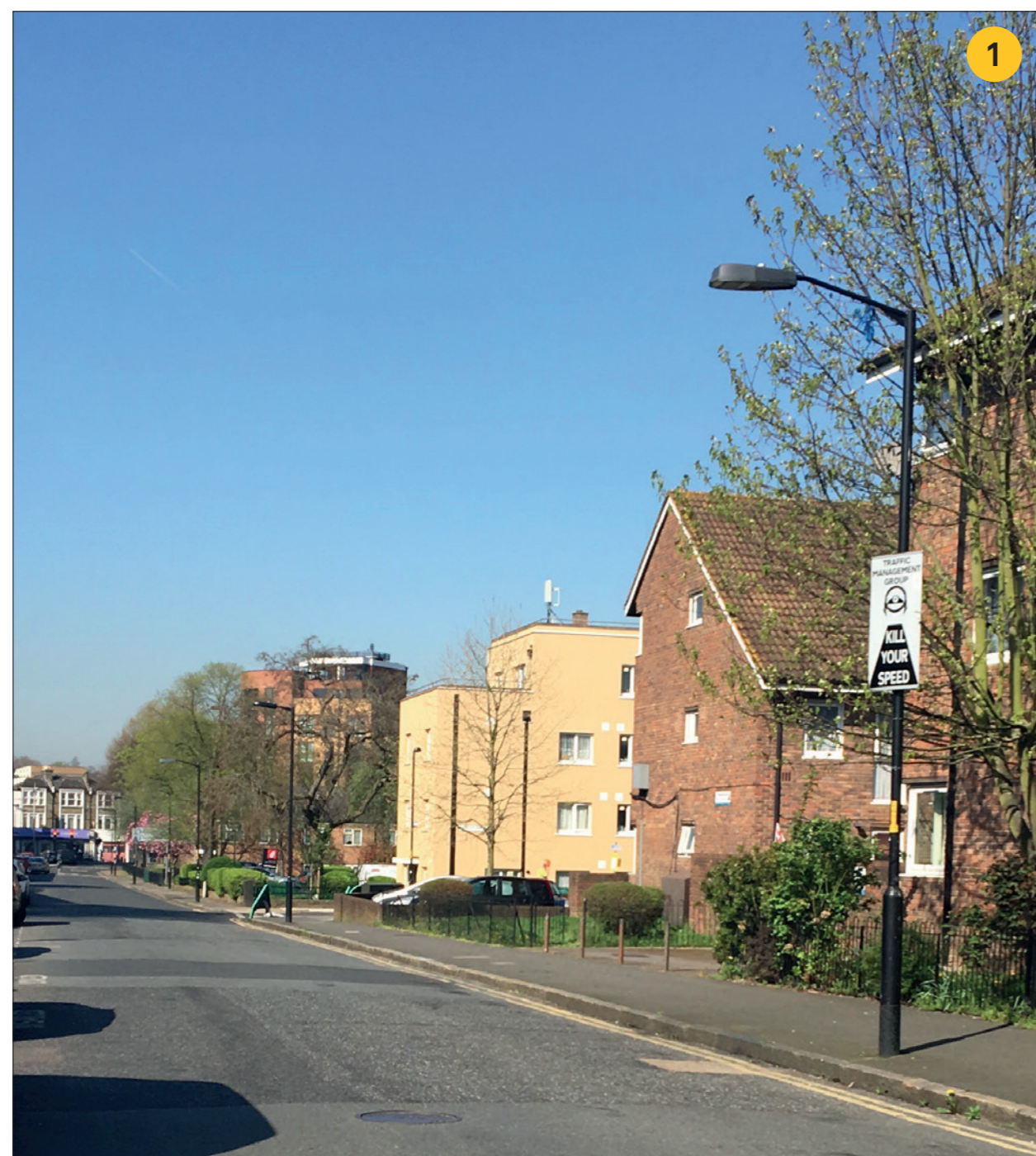
▲ View of site building from Heaton Road
