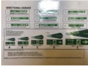
X-Fire exit signage 2018037.jpg
