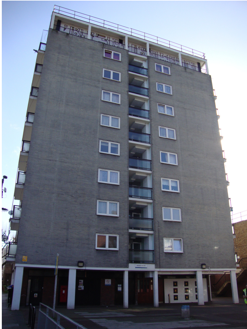
NAPIER HOUSE COOKS ROAD LONDON SE17
