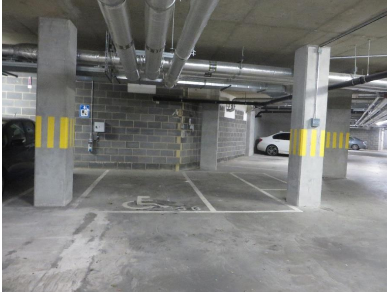
Figure 4.2: Disabled parking bays at site B
