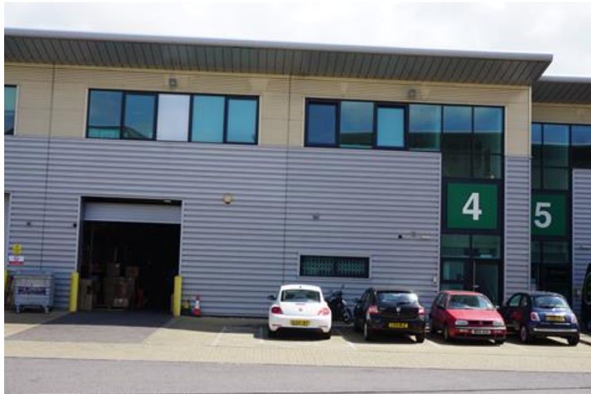
Figure 3.7 Example of relatively modern, replacement industrial stock
