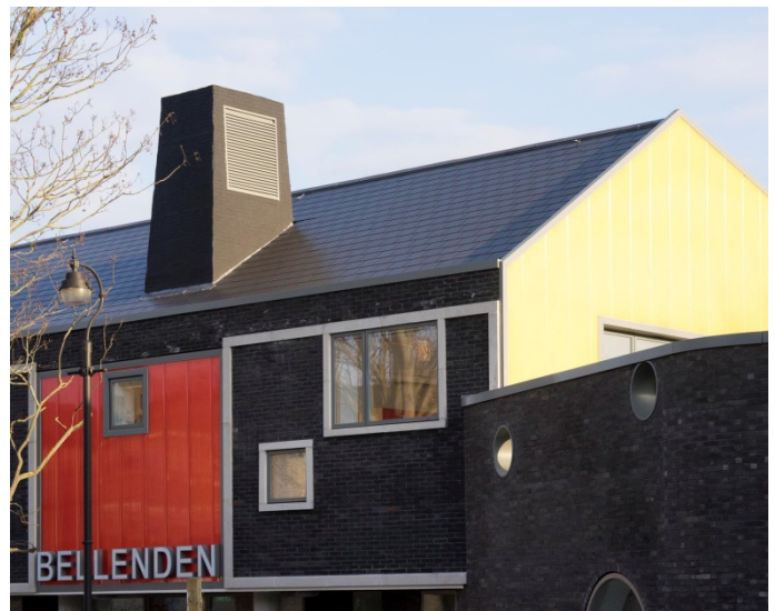
Bellenden School: Clear identity as a community beacon Cottrell & Vermeulen Architecture Photo by Anthony Coleman
