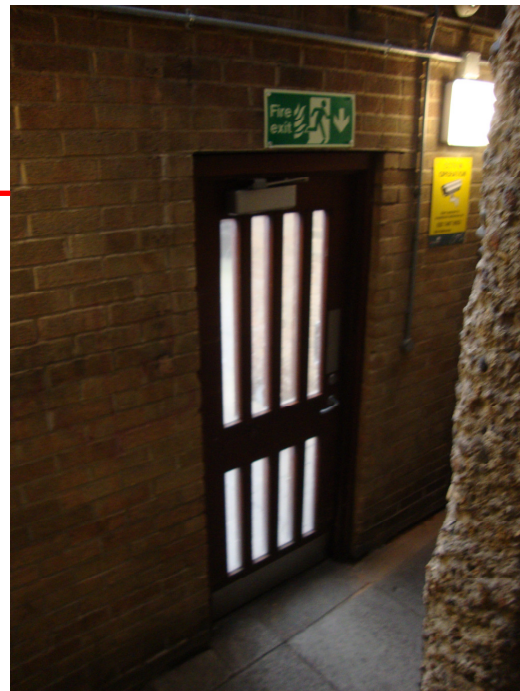
GROUND FLOOR EXIT DOOR
