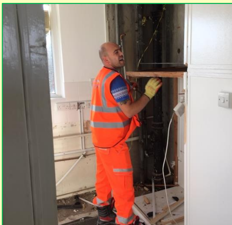
Pictured above is the stripping out of the
