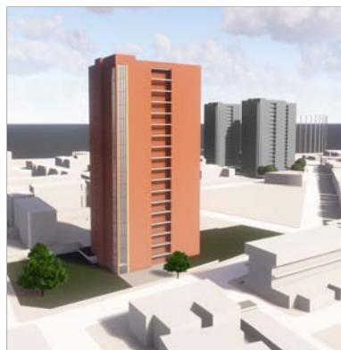
Aerial view from Junction between Ledbury Street and Commercial Way
